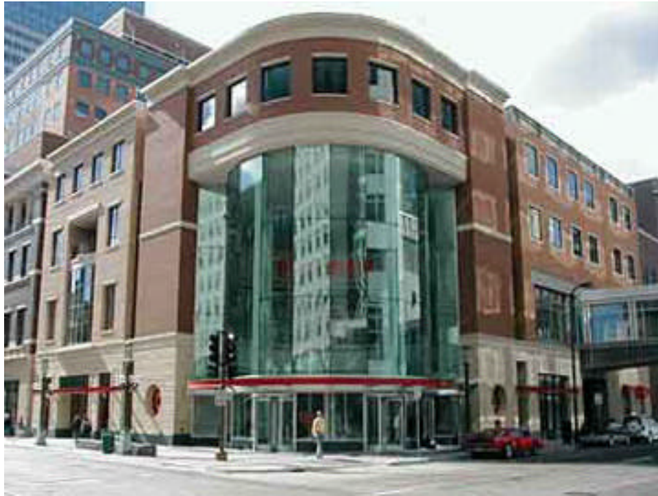
Exhibit 3: A Multi- Story Department Store in Minneapolis
